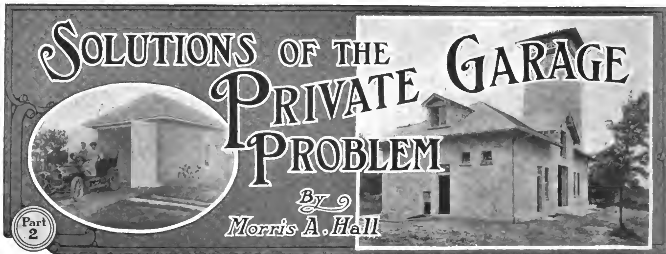
Of All Materials, Concrete Meets with the Most Favor—Two Types of Concrete Garages, One Small, One Large
